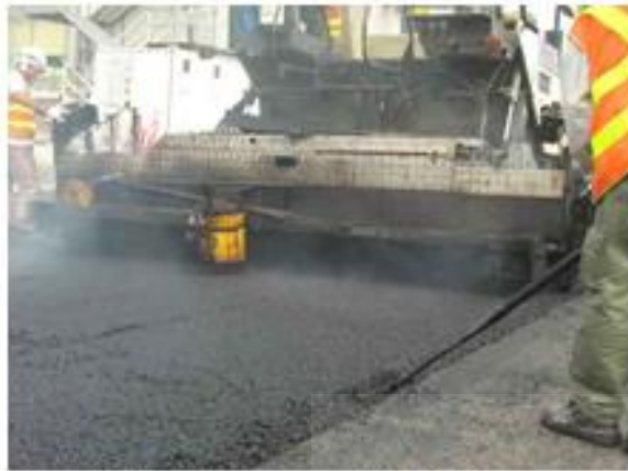
(a) Placement of AR Mixture
