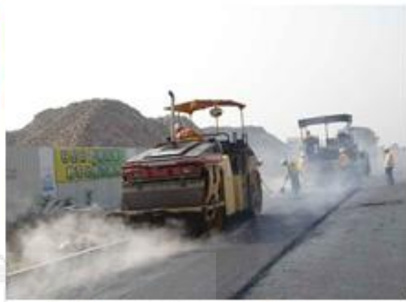
(b) Compaction of AR Pavement
