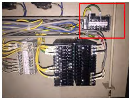
Setting ground terminal for SDC46.
