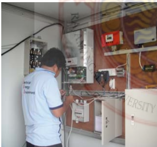
Figure.10: Installation of control and monitoring Unit
